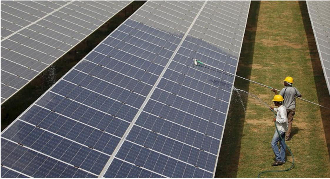
**Figure 8 – Example of cleaning of PV modules**
