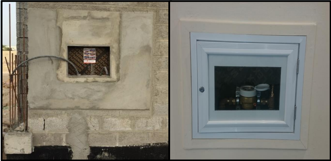
Figure 4. cavity Loop-in
