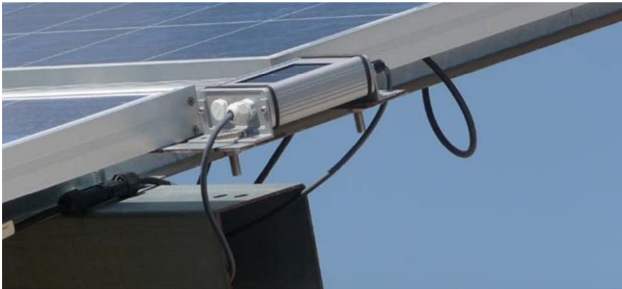
Figure 7 – Example of an in-plane PV sensor
