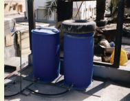
The height of ground storage tank is more than 1 meter which obstructs water to fill the tank
