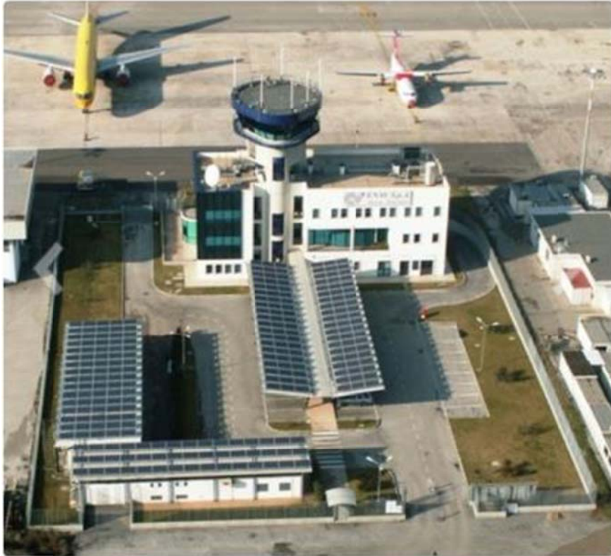
Figure 14 – PV plants in proximity of the tower within the Brindisi airport (source: ENAV website)
