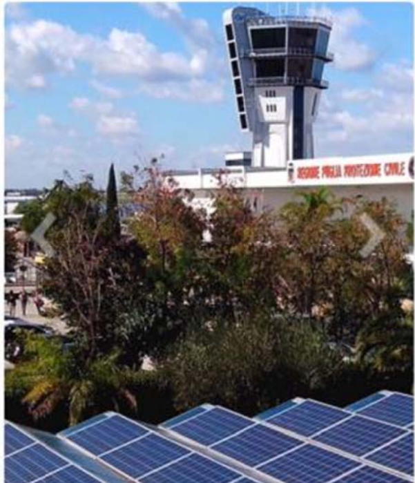
Figure 16 – PV plant on the rooftop of an operational buildings (source: ENAV website)
