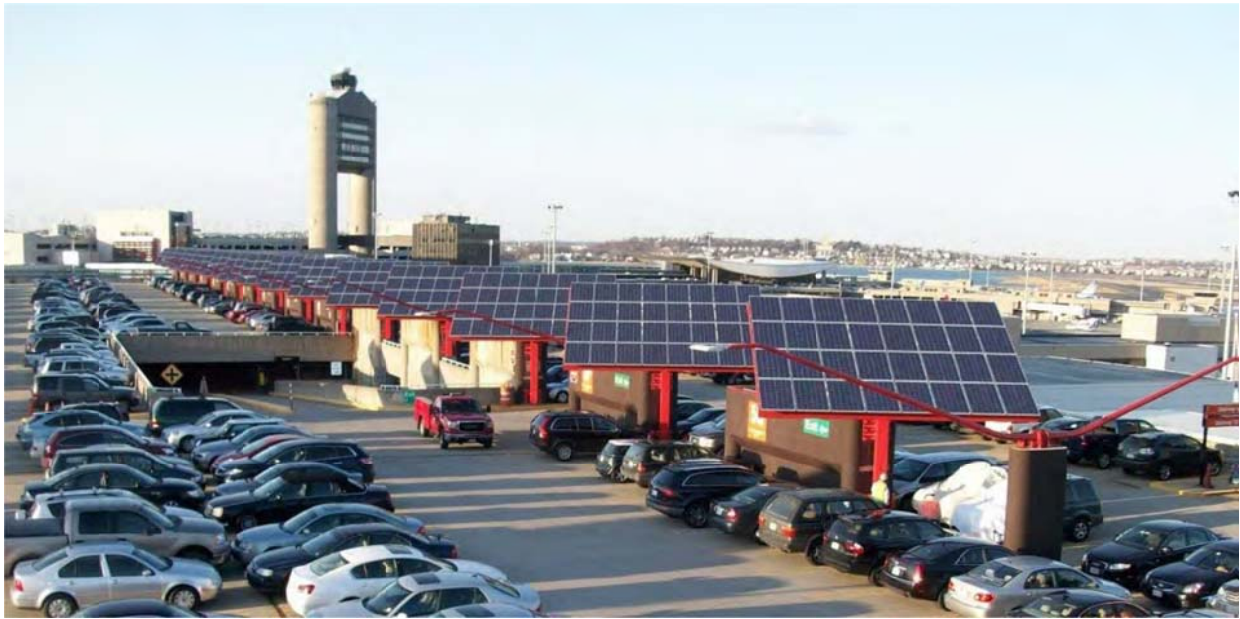
Figure 12 – Solar Trees on Parking Garage at Boston’s Logan Airport (source: [4])
